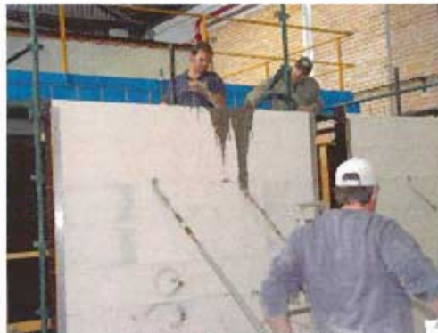
Concreting of 2.4m Square PanelForm with Minimum External Supports
